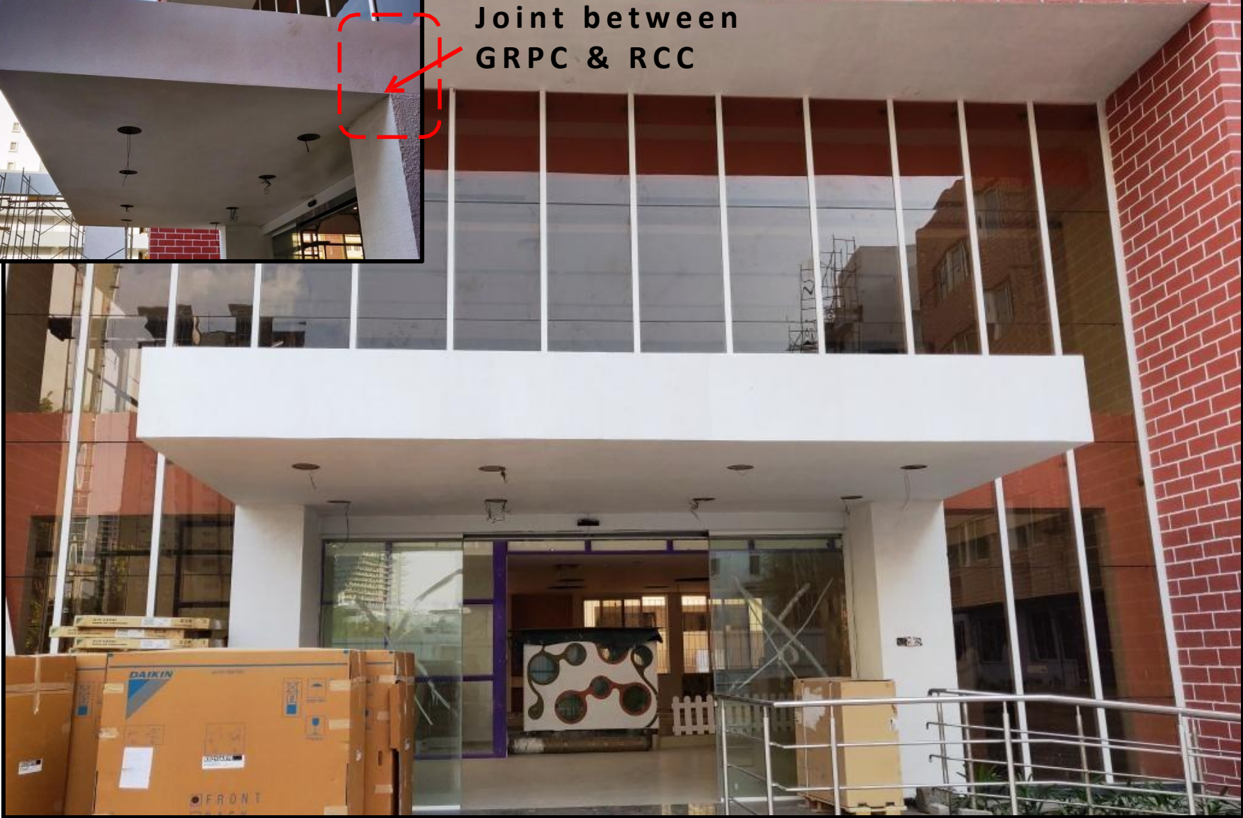
VASCON – AMENITY SCHOOL, PUNE– COMPOSITE CANTILLIVER CANOPY
